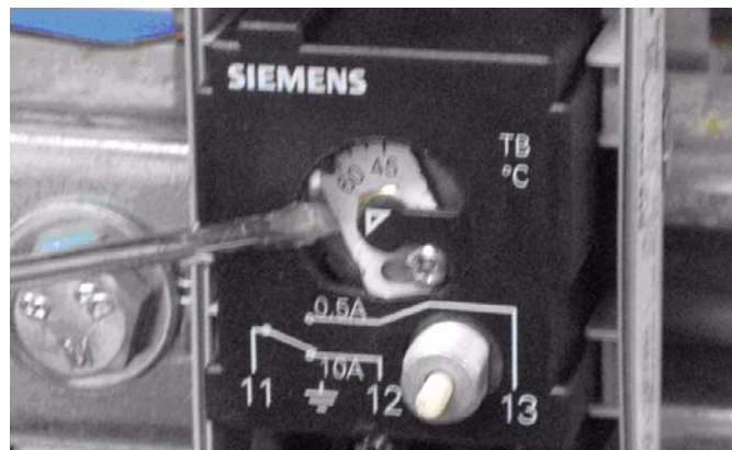
Figure 23 - Rotate Limit Thermostat Switch
