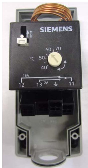
Figure 26 - Rotate adjustment on Limit Thermostat
