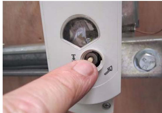
Figure 15 - Resetting Limit Thermostat
