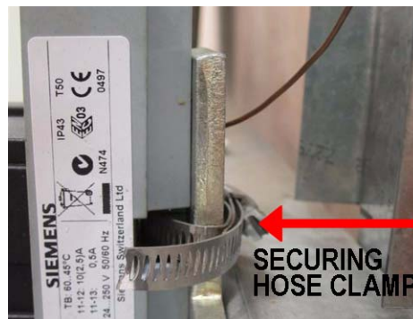
Figure 37 - Securing Hose Clamp
