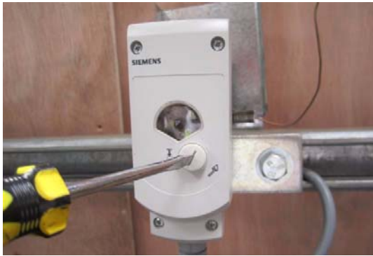
Figure 14 - Remove of Access Cover
