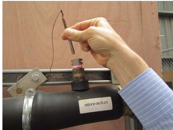
Figure 13 - Removal of Limit Thermostat Probe
