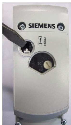
Figure 15a - Resetting Limit Thermostat
