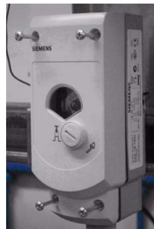
Figure 21 - Removal of Front Cover
